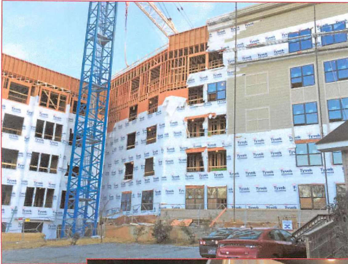
Figure 4 – View of a building in various stages of construction.
