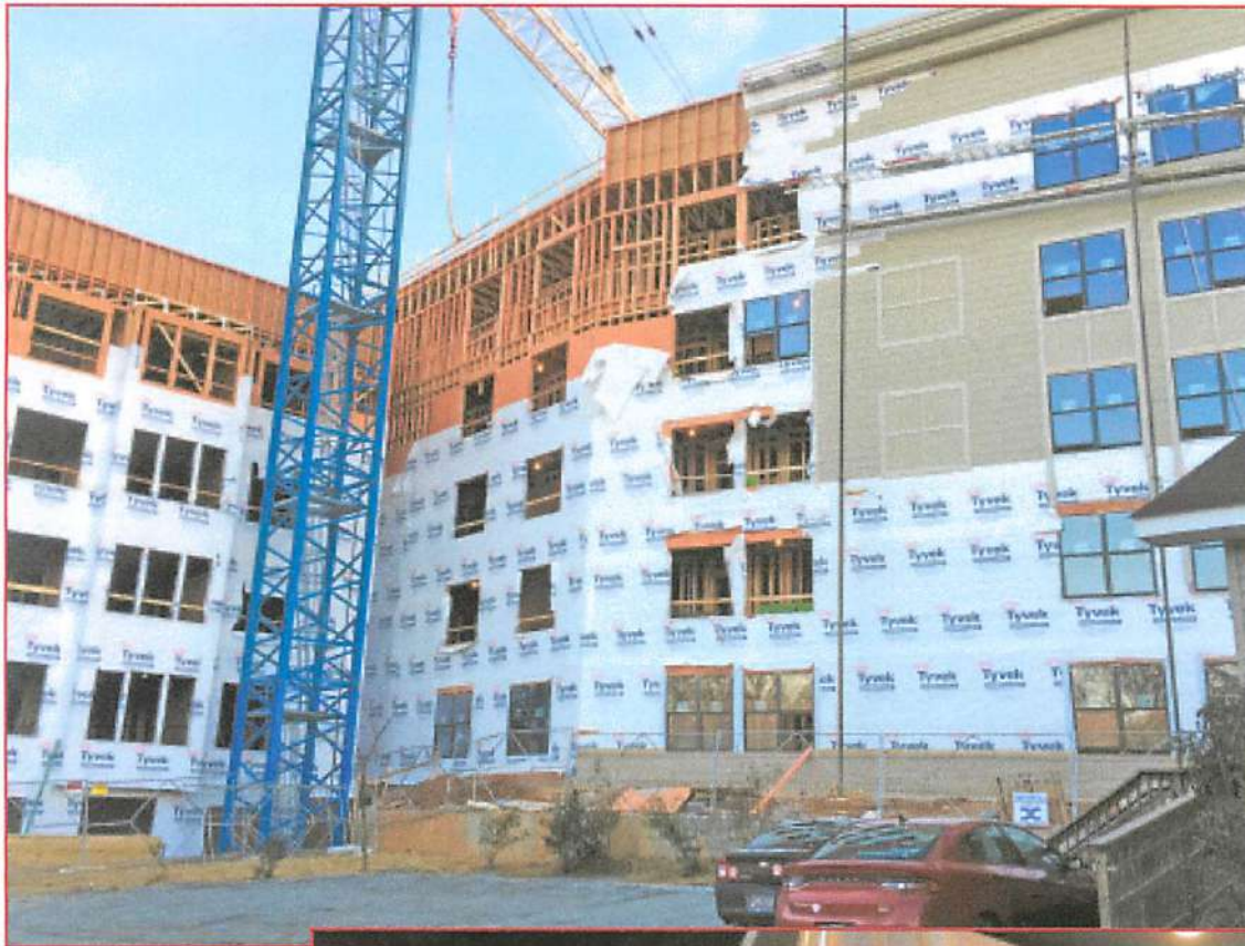
Figure 4 – View of a building in various stages of construction.
